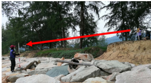
Figure 3: Total station survey execution
